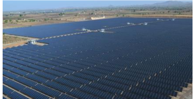
10MWp, free-field PV power plant, Rajkot, Gujarat
