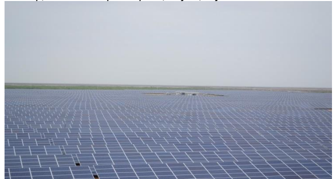
51MWp, free-field PV power plant, Charanka, Gujarat
